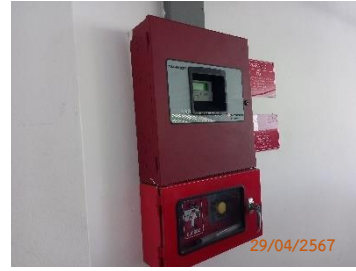
Fire Alarm Control Panel
