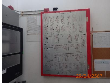
Graphic Annunciator Fire Alarm System
