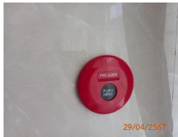
Fire Alarm Manual Station
